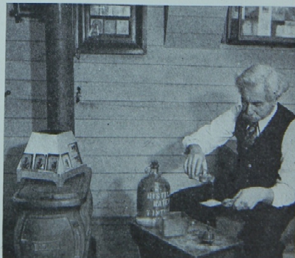
Fig. 7-1. Mr. C. H. Tremear of Greenfield Village, Michigan, shows how a Daguerreotype is made. Above: Buffing the plate, and testing the temperature of the mercury bath. Below: Exposing the plate, and gilding the Daguerreotype plate. (Courtesy Edison Institute.)
